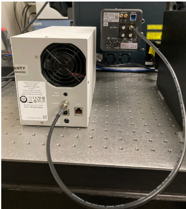
Figure 7. Cable connection from Timing 1 port of Hamamatsu ORCA-Fusion camera to SOLA light engine electronic shutter input.
